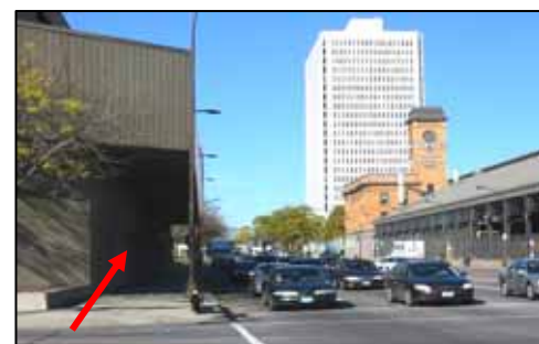
This sidewalk area on the Washington Avenue Commercial Corridor is dark and uninviting.
