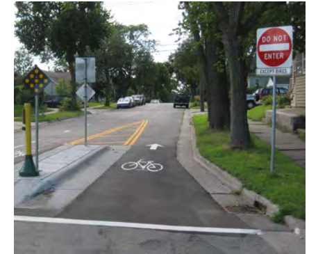
At some intersections, turning from or onto a bike boulevard is restricted for motorists.
