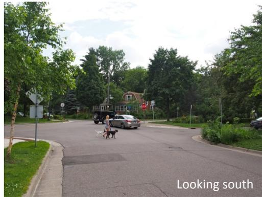
Due to the skewed intersection design, it is not always clear where approaching drivers on Bedford St SE should stop.
