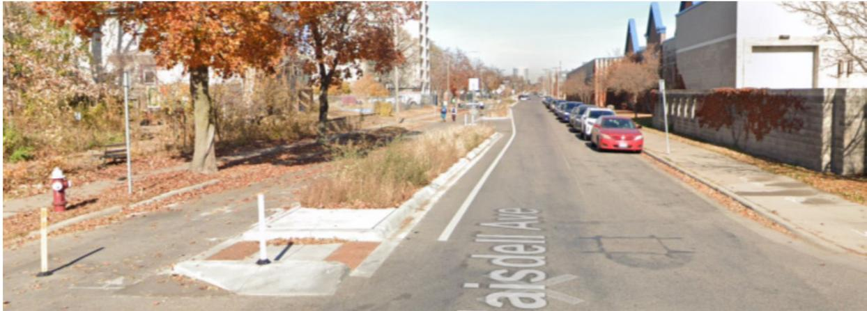
Figure 4: Example of a bikeway median/pedestrian safety island with greening
