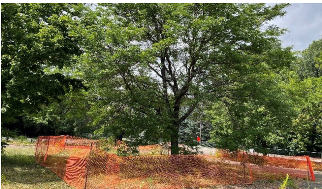
A large tree enclosed by an orange plastic mesh fence to protect it during construction activities.
