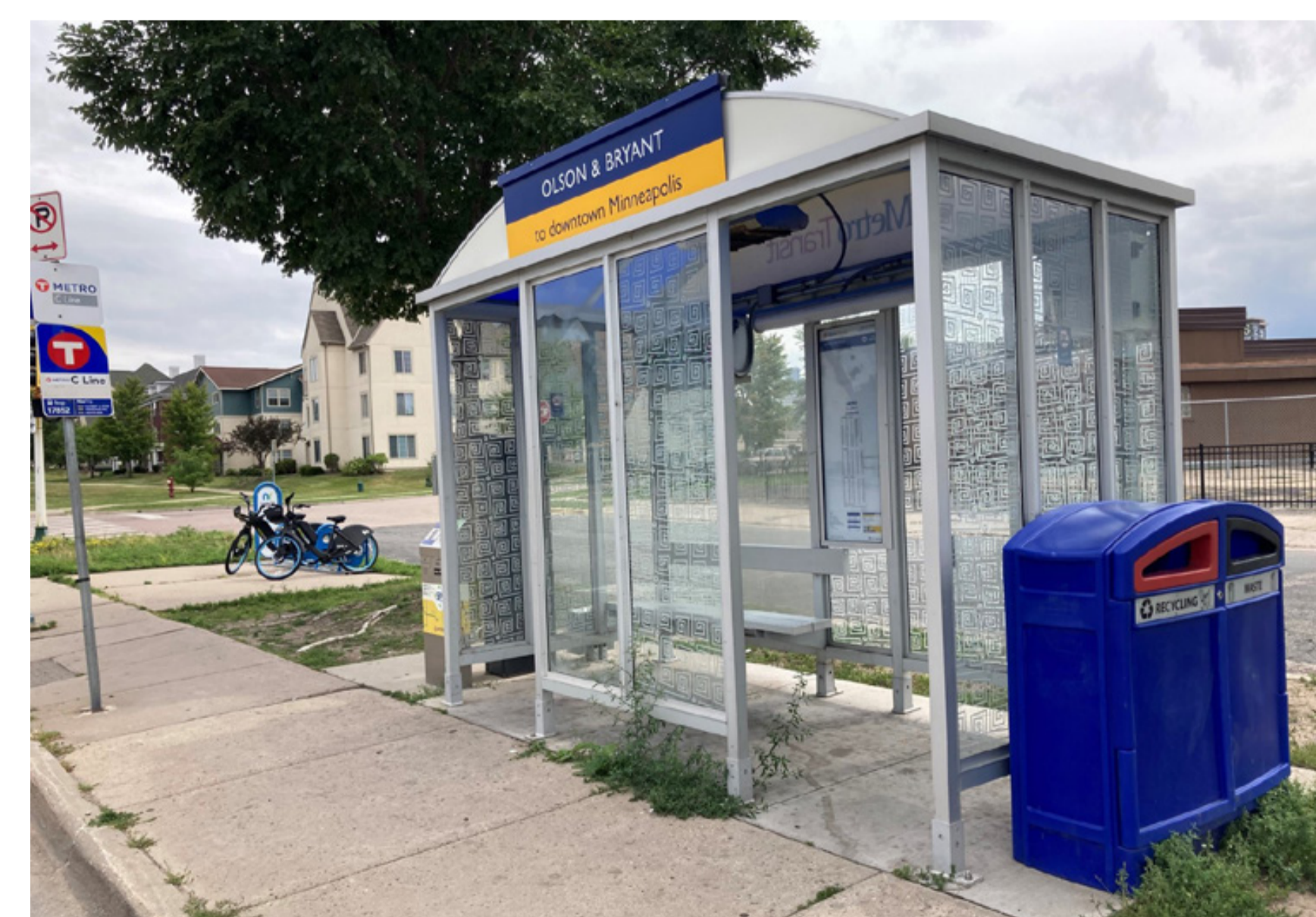
Example temporary station at Olson & Bryant for the C Line BRT route
