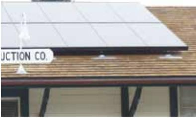
*Attach solar collectors to a historic roof in a minimally invasive and reversible manner. In this example the panels are mounted such that the original shingles are saved.*
