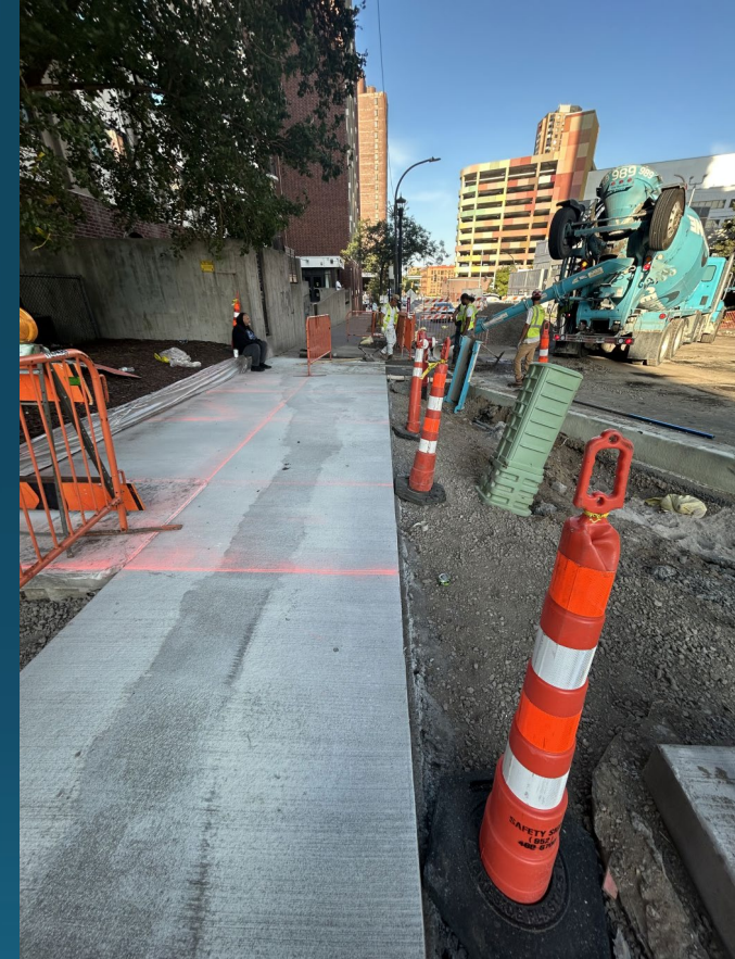
Grant St – Paving
