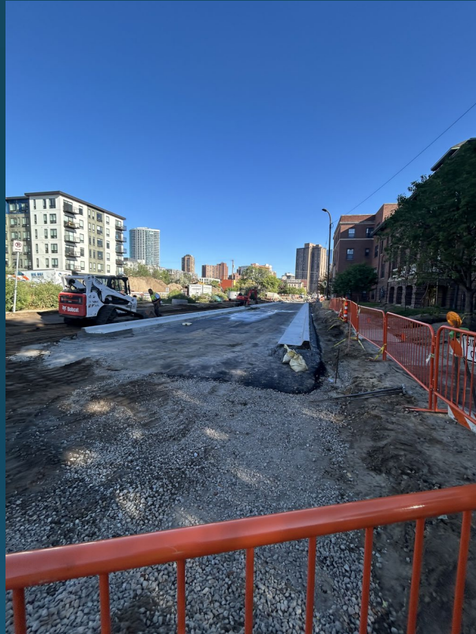
18 th St to 17 th St – Paving and Curb and Gutter
