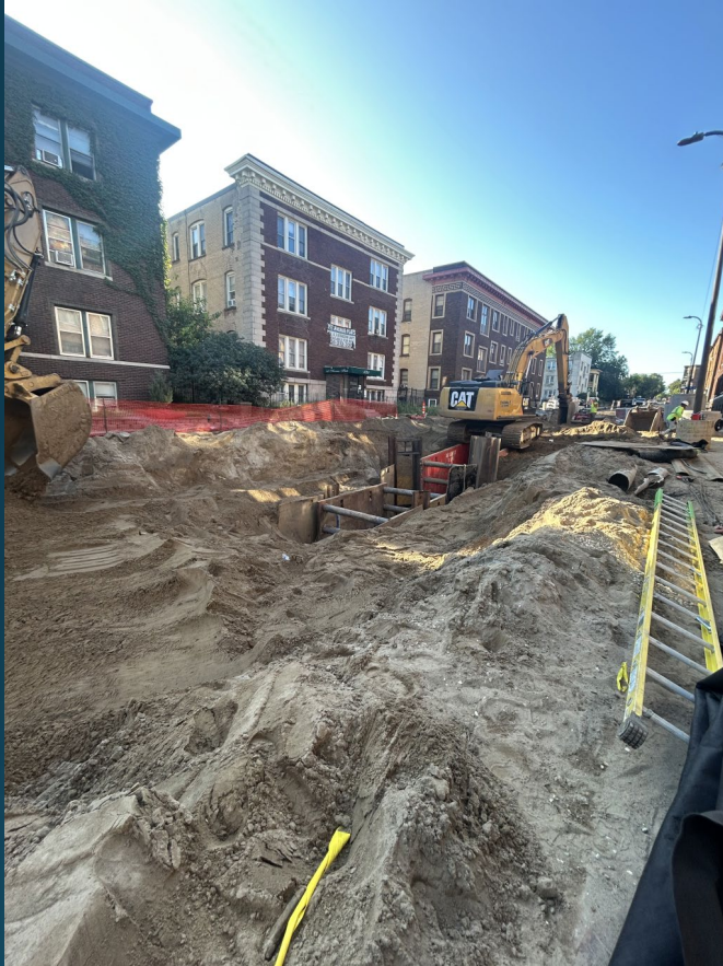
South of I-94 Bridge – Sanitary Installation
